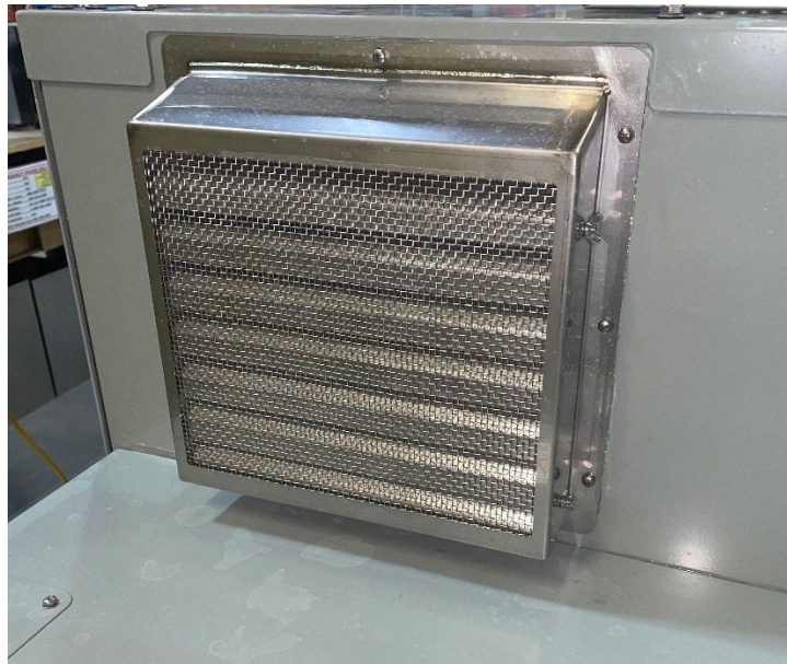
Figure 8-3 – Enclosure Intake Duct Screen
