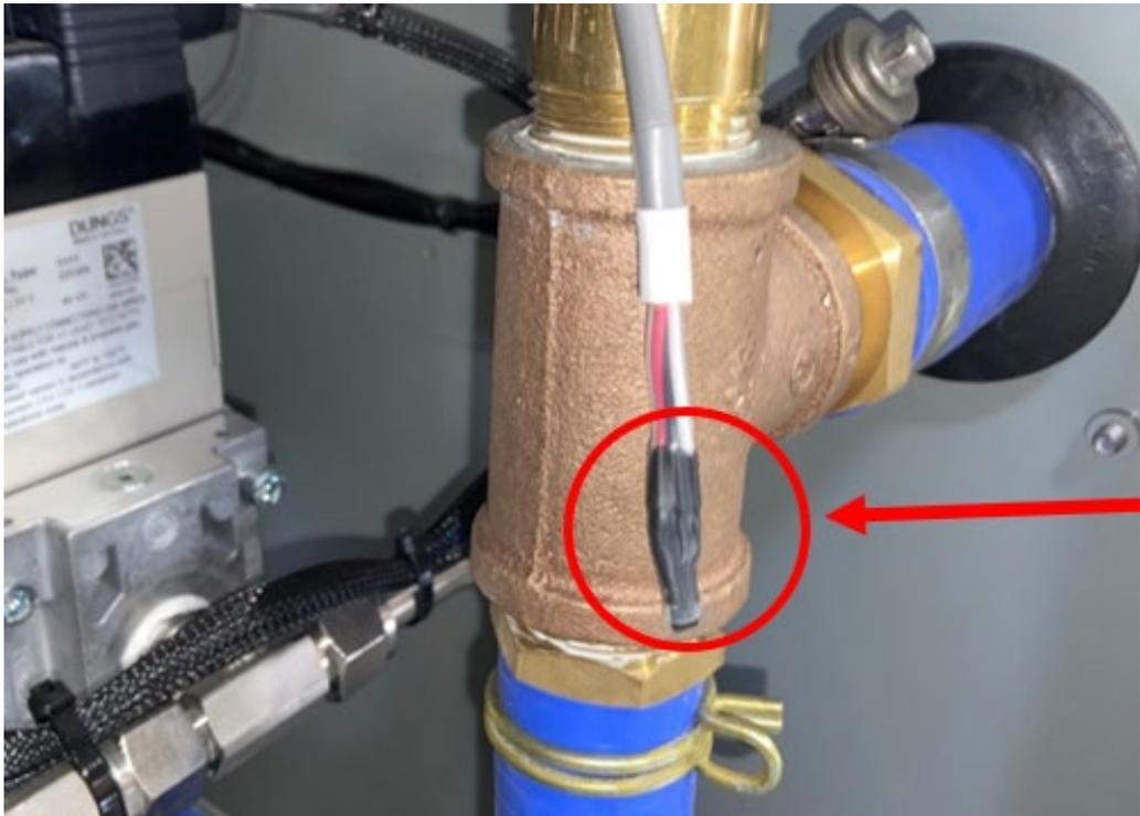
Figure 12-8 – #4 Radiator Inlet Temperature Sensor
