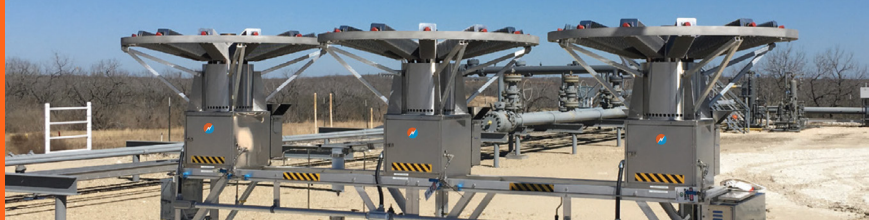
1500 watt Auto-CP system on natural gas pipeline, Texas, USA
